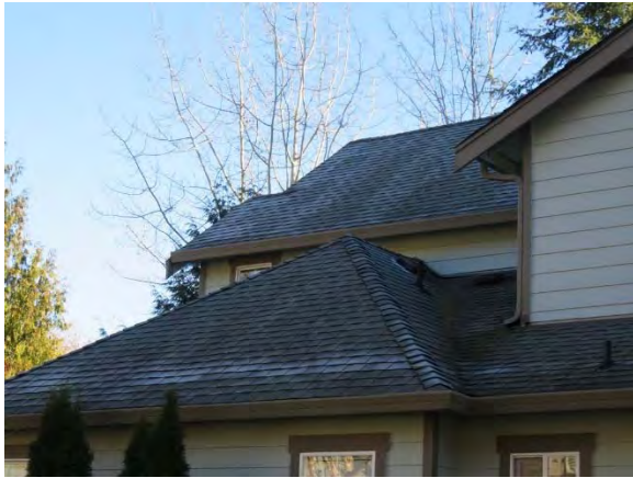
Typical Roof Surface
