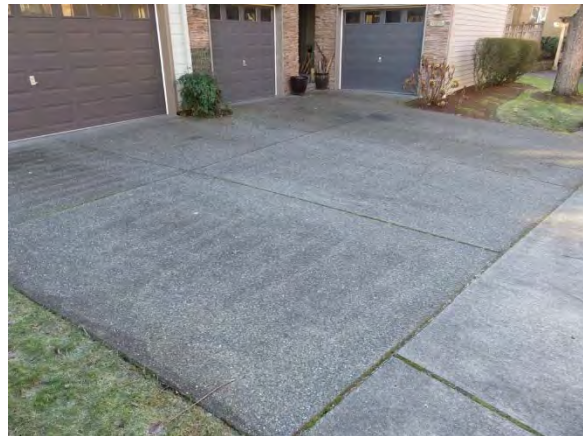
Typical Concrete Aggregate Driveway
