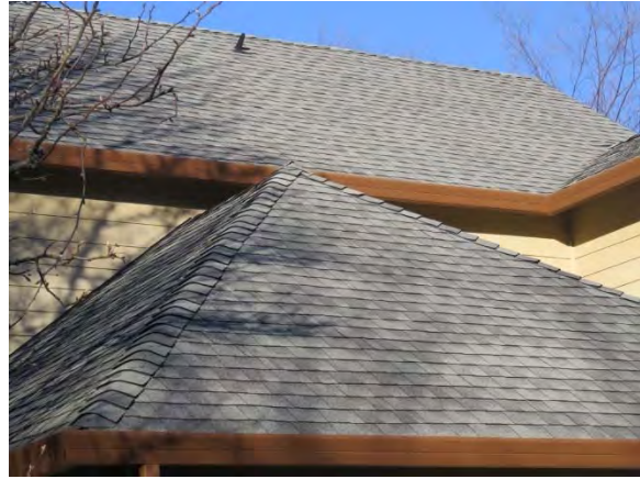
Typical Roof Surface
