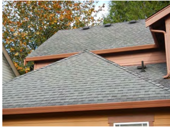
Typical Roof Surface
