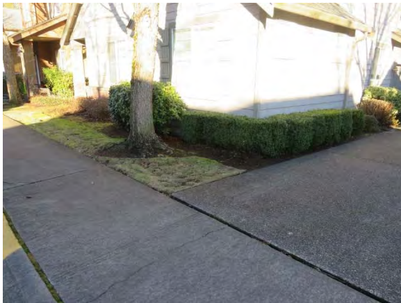
Typical Sidewalk and Driveway Trip Hazard
