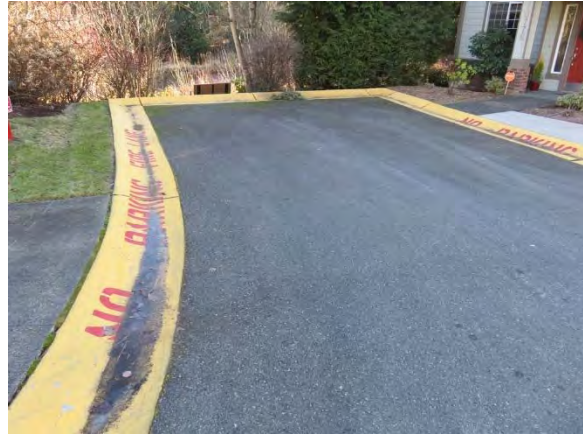
Typical Extruded Concrete Curb
