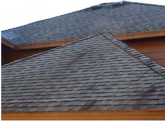
Typical Roof Surface
