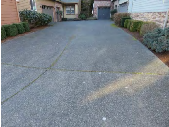
Typical Concrete Aggregate Driveway
